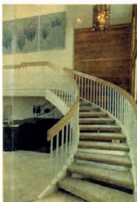
Suspended stairway in the home of Mr. and Mrs. Richard Long is supported only at the top and bottom. ↑ TH13
